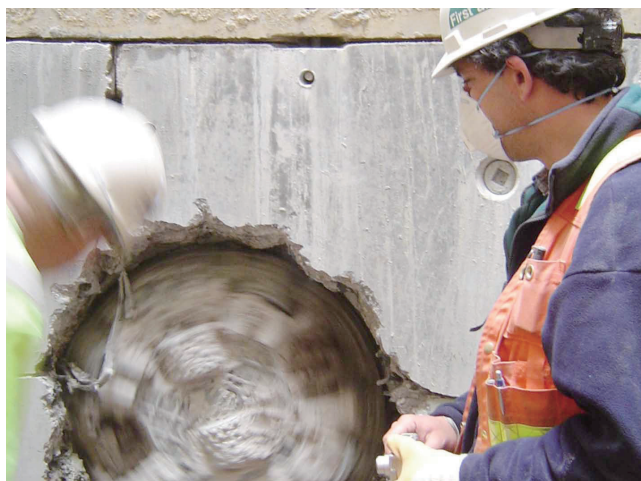
UNCLEMOLE SUPER AFTER COMPLETING A DRIVE THROUGH HARD ROCK
